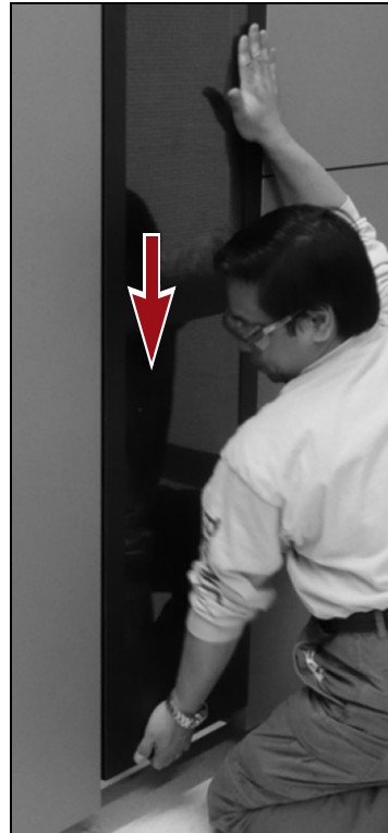
Figure 39 Slide the panel down into place.
