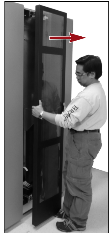
Figure 5 Lift the panel out and away from the frame.
