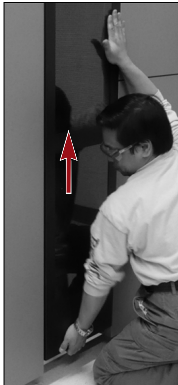
Figure 4 Slide the panel up to disengage the hangers.
