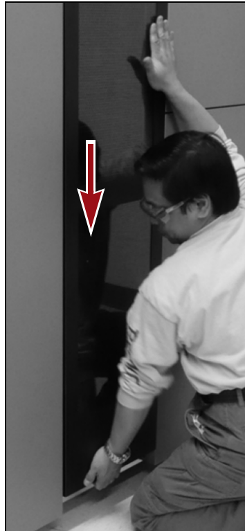
Figure 48 Slide the panel down into place.
