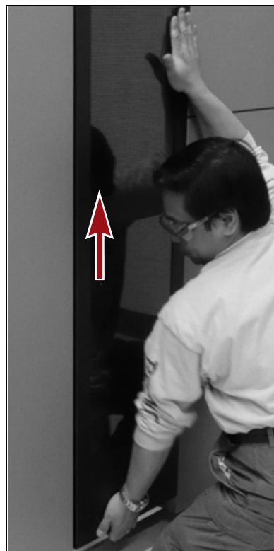
Figure 8 Slide the panel up to disengage the hangers.
