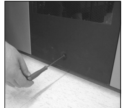
Figure 49 Install the screw to secure the panel.
