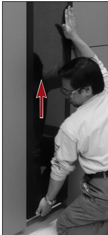
Figure 8 Slide the panel up to disengage the hangers.
