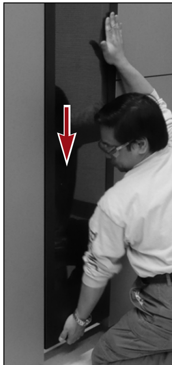
Figure 37 Slide the panel down into place.
