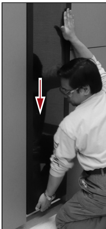
Figure 73 Slide the panel down into place while holding it steady higher up.
