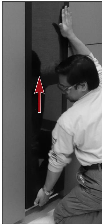
**Figure 10** Slide the panel up to disengage the hangers.
