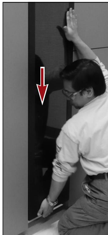
**Figure 37** Slide the panel down into place.
