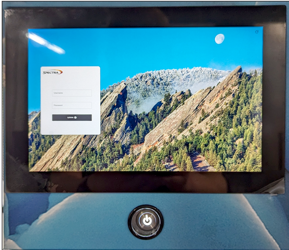
Figure 4 The library operator panel touch screen displaying the Dashboard of the LumOS user interface.
